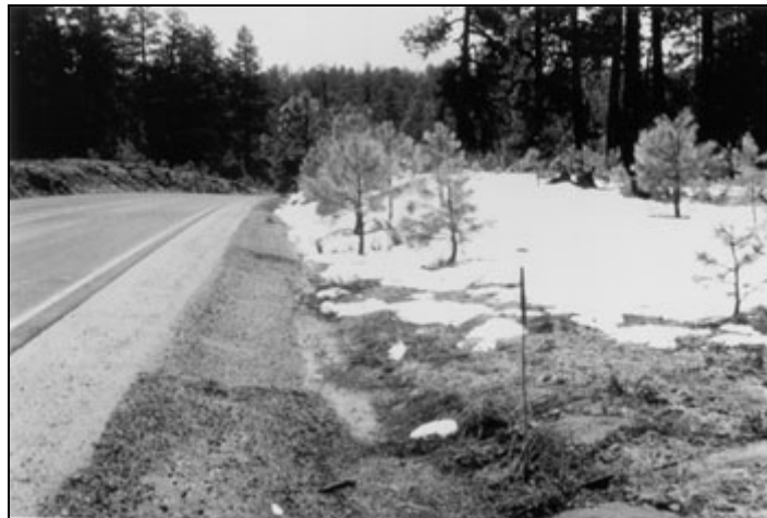
Clear zone about 10 ft; sideslope about 1V:3H, marginally recoverable.
