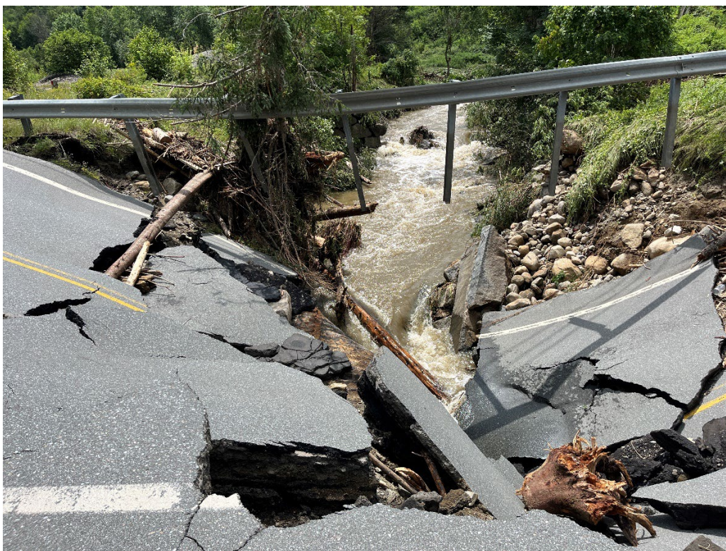
FIGURE 6-1 PAVEMENT WASHOUT AND ROAD COLLAPSE FROM RIVERINE FLOODING
