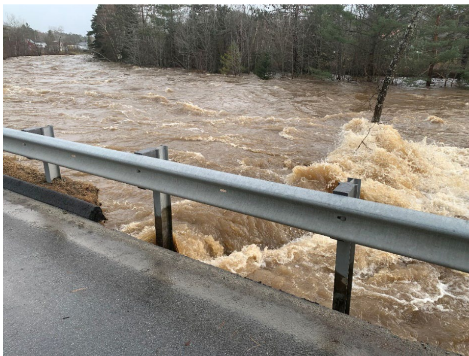
FIGURE 8-1 BRIDGE NEARLY OVERTOPPING FROM FLASH FLOODING
