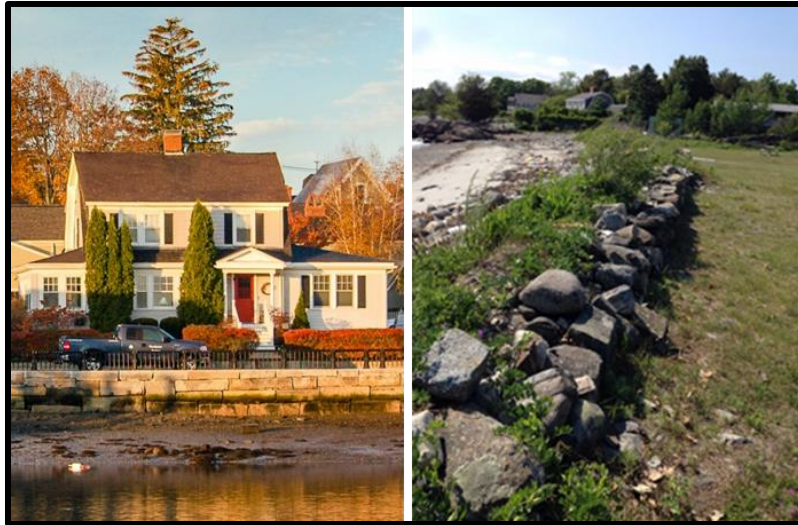
Figure 5: The image on the left is an example of a seawall, while the image on the right is an example of a rock wall.
