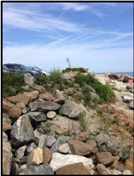
Figure 3: Example of a rip rap structure.
