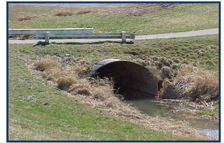
Before Mitigation and After Mitigation
