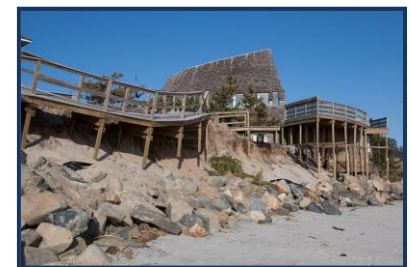
Severe beach erosion and damage resulting from a nor’easter.
