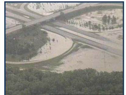
When large highways close due to flooding, traffic is detoured causing inconvenience and economic loss.
