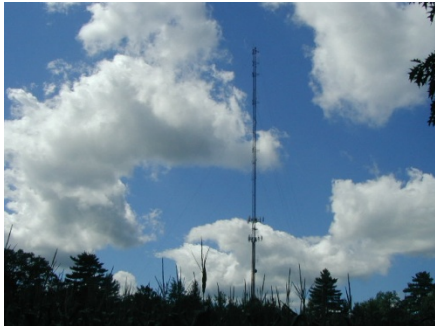
Figure 34: Hoyt Cell Tower, Town of Chester
